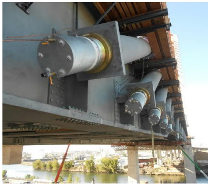
Figure 6 – Phase 2 Main Span Lower Cable Connection
