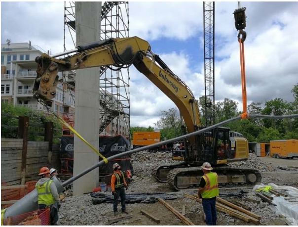
Fig. 7.1. Tie Down cable installation
