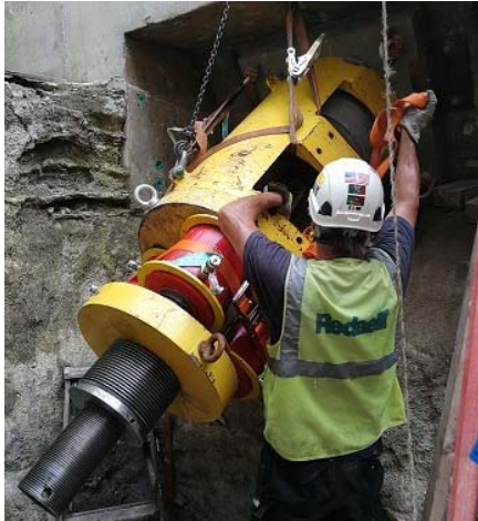
Fig. 7.7. Tie Down cable tensioning
