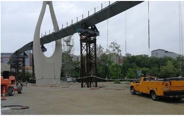
Fig. 8.1. Main cable temporarily lifted
