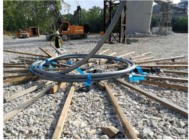
Fig. 7.2. Uncoiling Main cable
