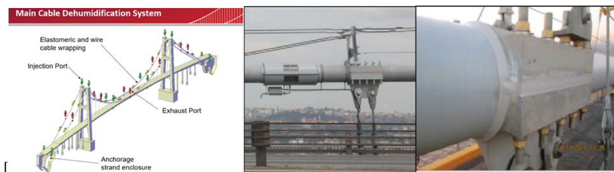
Figure 7: Dry air injection and exhaust port locations and air-tight elastomeric wrapping /sealing
