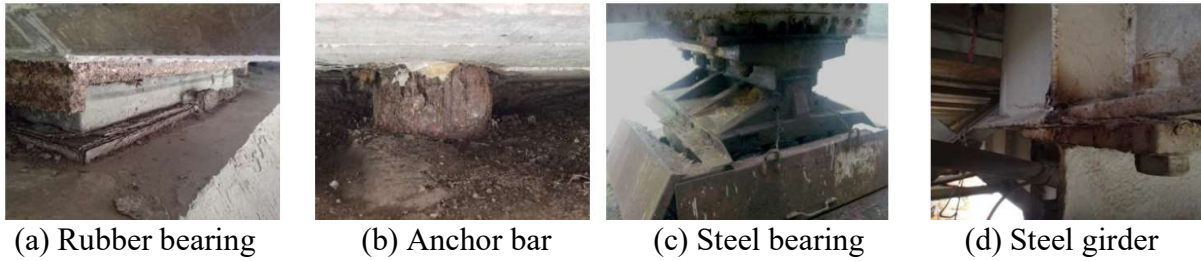
Figure 1: Corrosion Damage in Bridge Bearings Installation Area
