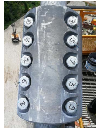
Fig. 7.4. Clamps installed on Main cable
