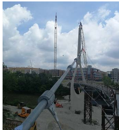
Fig. 7.6. Hangers connected loosely
