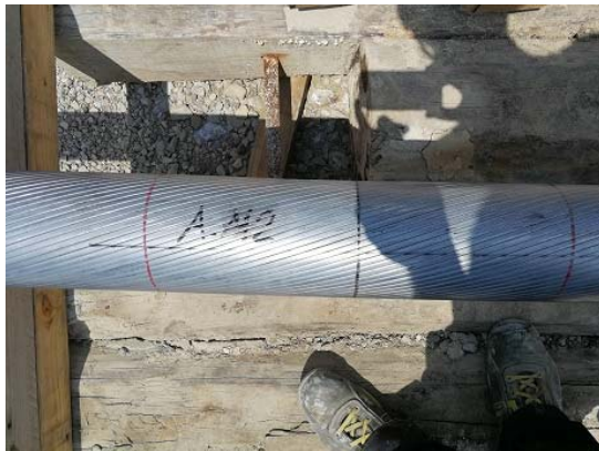
Fig. 7.3. Marking for clamps positioning
