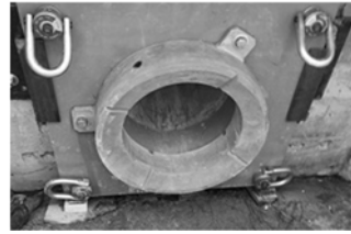
Fig. 4.8. Photo of Spherical washer installed
