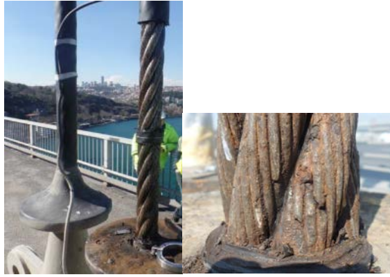
Figure 10: Polyethylene sheath and trumpet (left) and the flat top surface of the lower socket (right)
