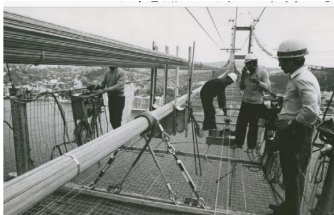
Figure 3: Original cable construction of the first Bosphorus Bridge using the arial spinning method
