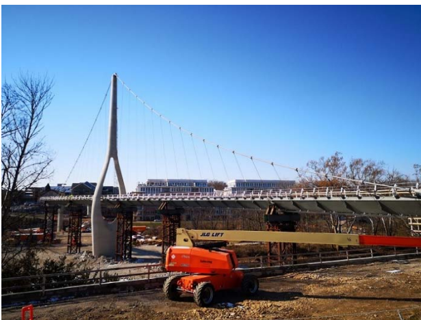
Fig. 9.1. Bridge at end of tensioning
