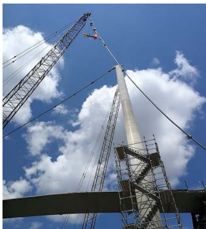
Fig. 7.5. Main cable installation to the mast
